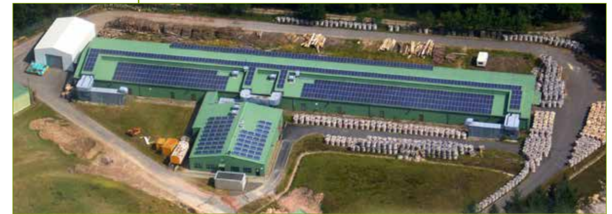
Subarea storage building and other offices (developed)
