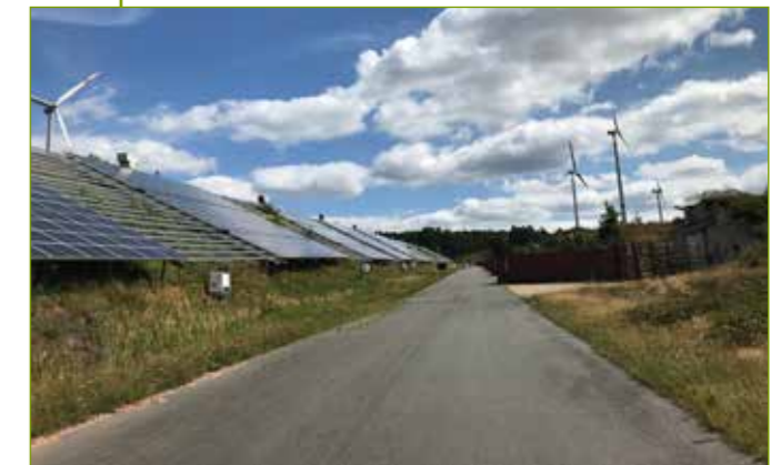
2.3 MW PV system on a backfilled bunker row
