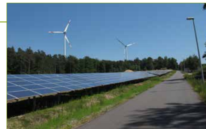
Access road "Solar-Allee" inside the developed area
