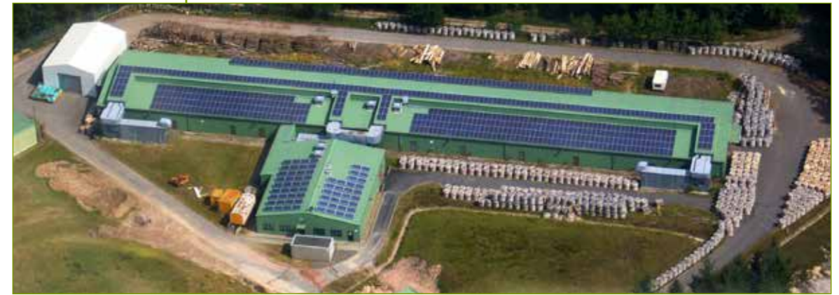
Subarea storage building and other offices (developed)
